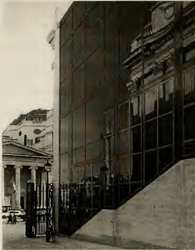
Fig. 4.6 – Exterior view of glass-walled grand stair.
